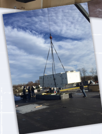
A giant crane lifts a rooftop air handling unit for placement on WEMOCO.
